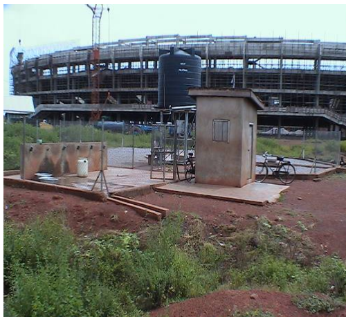
Rehabilitated System with the New Tamale Sports Stadium Construction in the background
